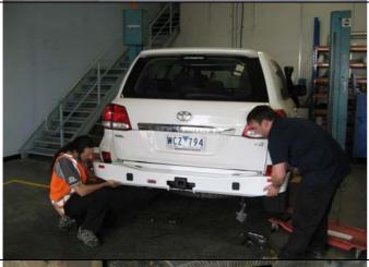
15. With the help of another person place bar gently on vehicle and secure loosely with original tie down bolts.
